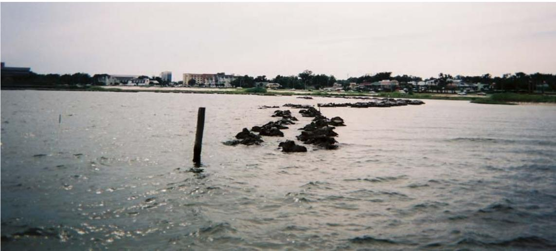
Figure 5. Wave propagation through the gap between the structure and the seawall (below the bottom of the picture). Note the reflected waves propagating nearly parallel to the structure.
